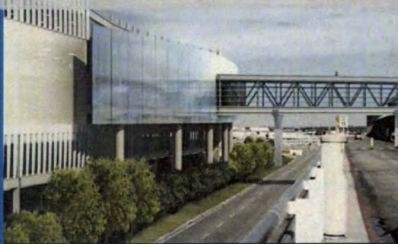
Consolidated Rental Car Facility (CONRAC)
