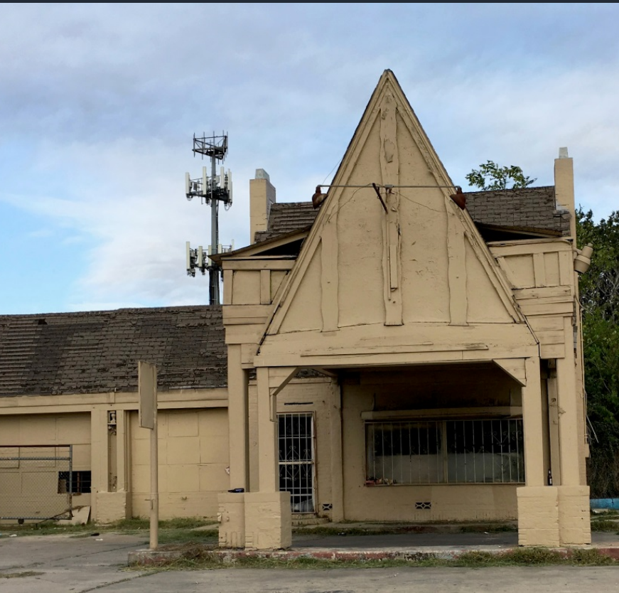
Gas station structure: contributing
