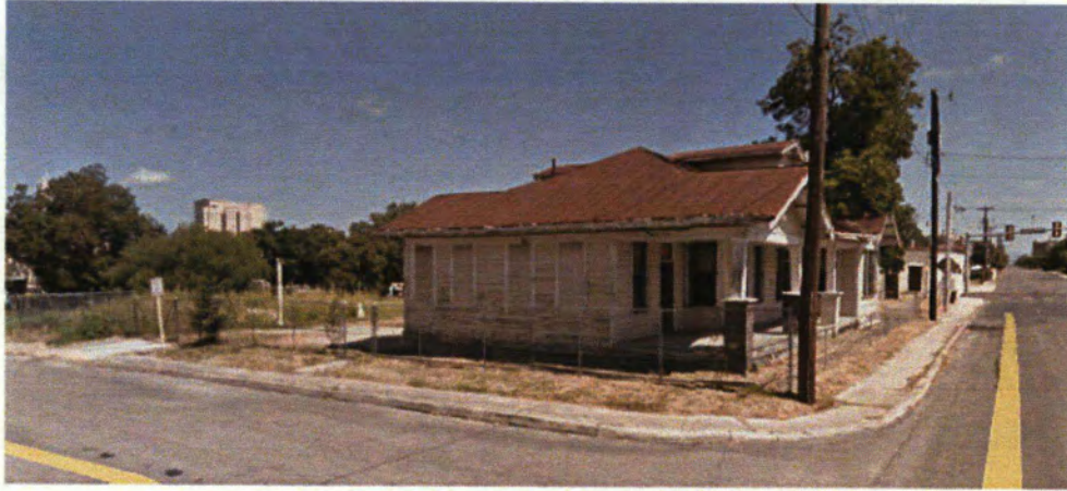
Residential structure located in the rear of 1434 E. Commerce parcel on the corner of Hackberry and Idaho.
