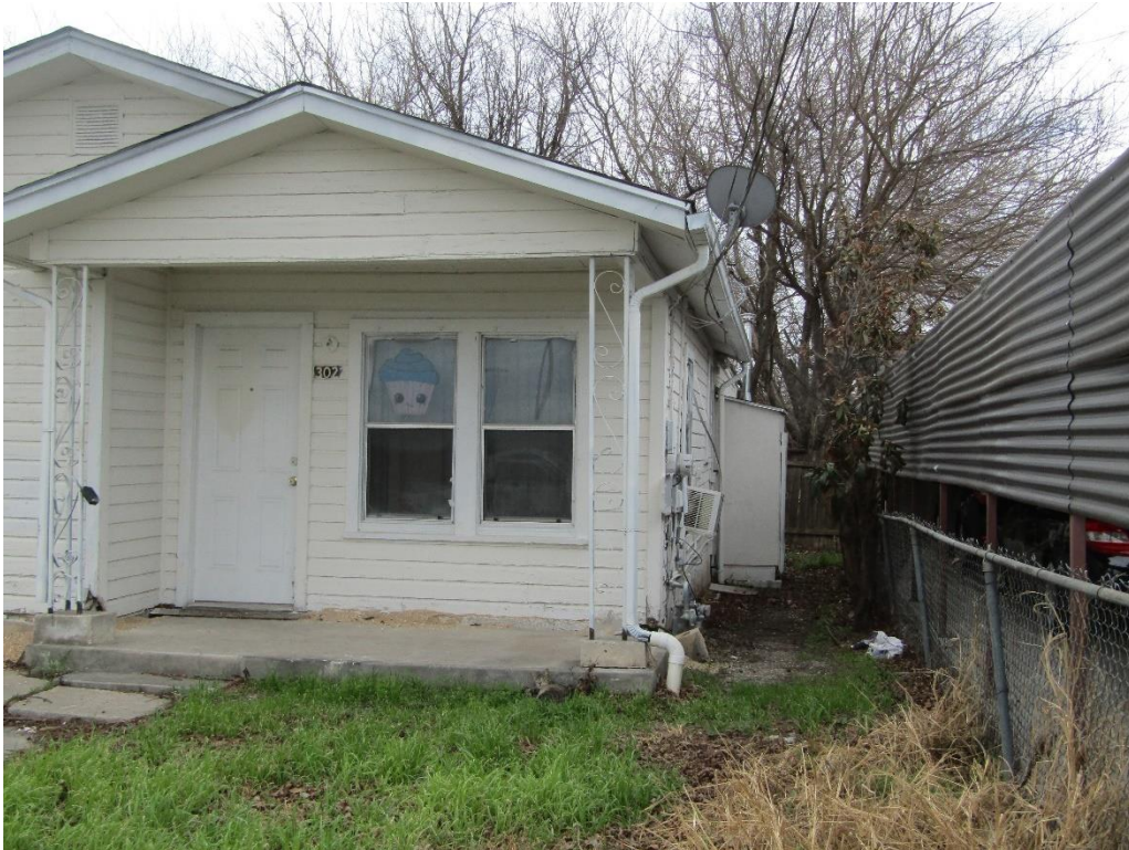
Subject Property (Water Heater proximity to side property line)
