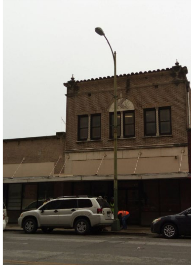
LOOKING W AT SUBJECT SITE
