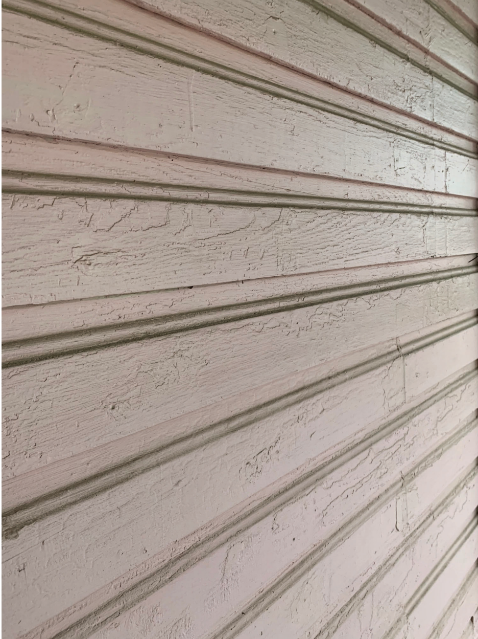
Existing Wood Siding
