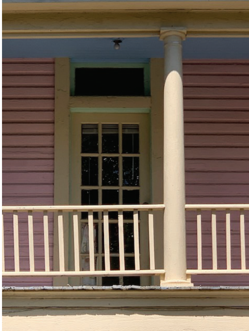
Existing Second Floor Porch Wood Railing
