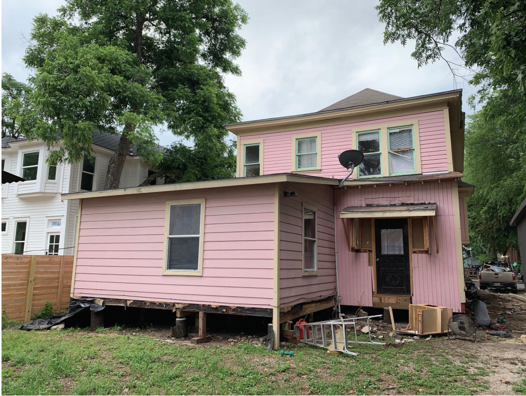
Rear of House (East Facing)
