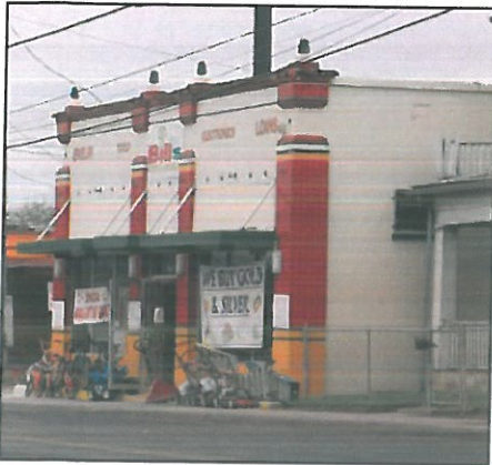
Commercial Building 105 S. Zarzamora
