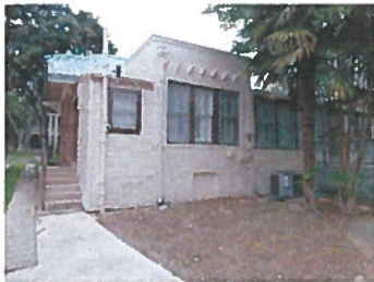
PHOTO 2 - REAR OF HOUSE
