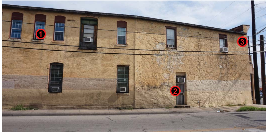
② ORIGINAL OPENINGS TO REMAIN. DETERIORATING NON-ORIGINAL WINDOWS AND DOORS TO BE REPLACED
