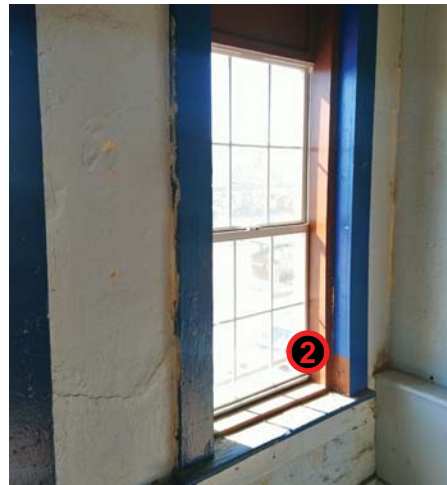
② EXISTING NON-ORIGINAL WINDOW. VIEW FROM INSIDE. NON-ORIGINAL WINDOWS FRAMED INSIDE ORIGINAL OPENING
