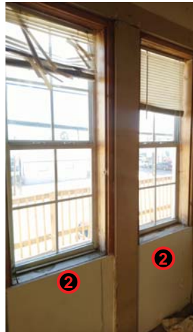
② EXISTING NON-ORIGINAL WINDOW. VIEW FROM INSIDE. NON-ORIGINAL WINDOWS FRAMED INSIDE ORIGINAL OPENING
