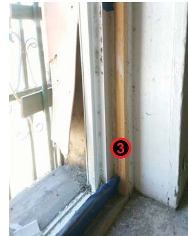
3 EXISTING NON-ORIGINAL WINDOW. CLOSER VIEW FROM INSIDE OF NON-ORIGINAL WOOD SASH
