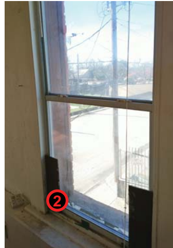
2 EXISTING NON-ORIGINAL WINDOW. VIEW FROM INSIDE. NON-ORIGINAL WINDOWS FRAMED INSIDE ORIGINAL OPENING
