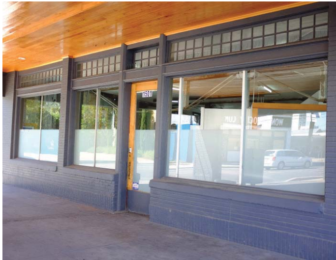
G EXHIBIT G NON-HISTORIC ALUMINUM STOREFRONT W/ FROSTED FILM ON EXISTING STOREFRONT OPENING
