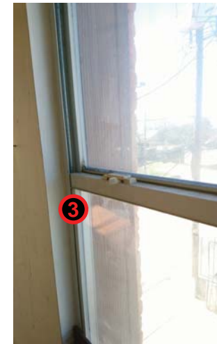
3 EXISTING NON-ORIGINAL WINDOW. CLOSER VIEW FROM INSIDE OF NON-ORIGINAL WOOD SASH
