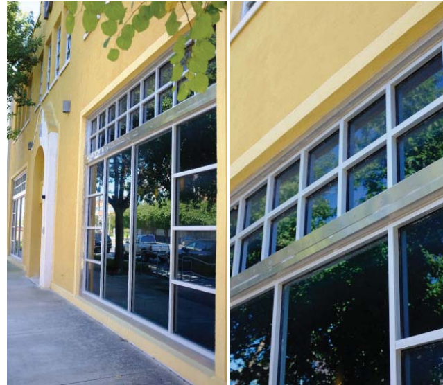
D EXHIBIT D NON-HISTORIC ALUMINUM STOREFRONT W/ TINTED GLASS ON EXISTING OPENING
