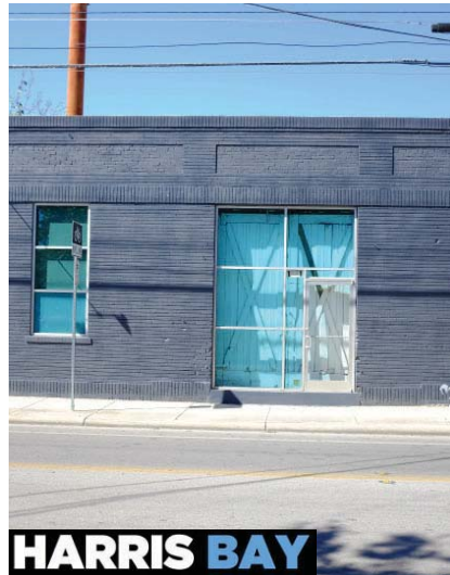
F EXHIBIT F PAINTED BRICK FACADE AND NON- HISTORIC ALUMINUM STOREFRONT ON EXISTING OPENINGS
