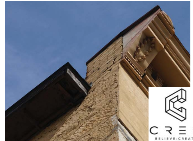
③ EXISTING ROOF TO BE ASSESSED AND REPAIRED/REPLACED AS NEEDED. CORNICE TO REMAIN AND TO BE REPAIRED.
