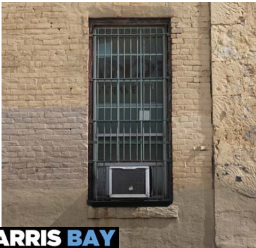
1 EXISTING NON-ORIGINAL WINDOW. NON-ORIGINAL WINDOWS ARE INSTALLED THROUGHOUT THE ENTIRE BUILDING
