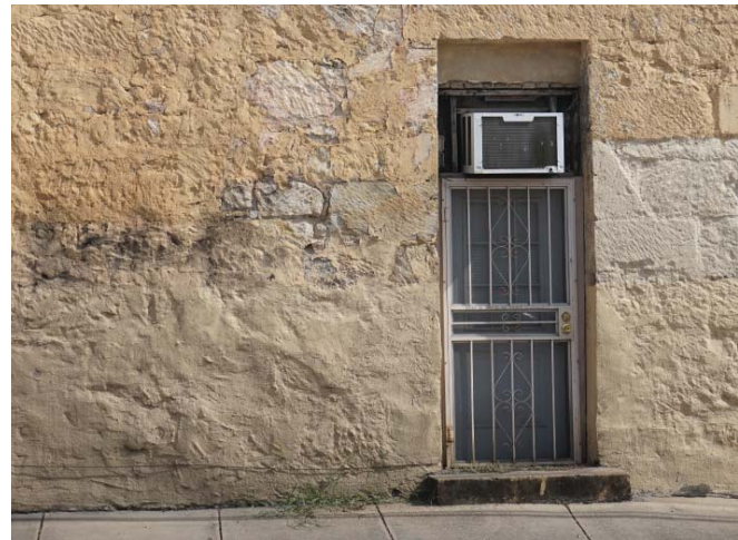
② ORIGINAL OPENINGS TO REMAIN. DETERIORATING NON-ORIGINAL WINDOWS AND DOORS TO BE REPLACED
