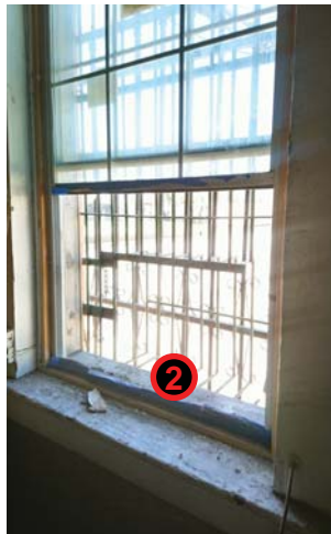
2 EXISTING NON-ORIGINAL WINDOW. VIEW FROM INSIDE. NON-ORIGINAL WINDOWS FRAMED INSIDE ORIGINAL OPENING
