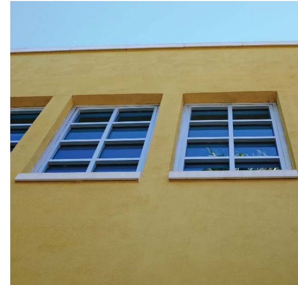
E EXHIBIT E NON-HISTORIC ALUMINUM WINDOWS W/ TINTED GLASS ON EXISTING OPENING
