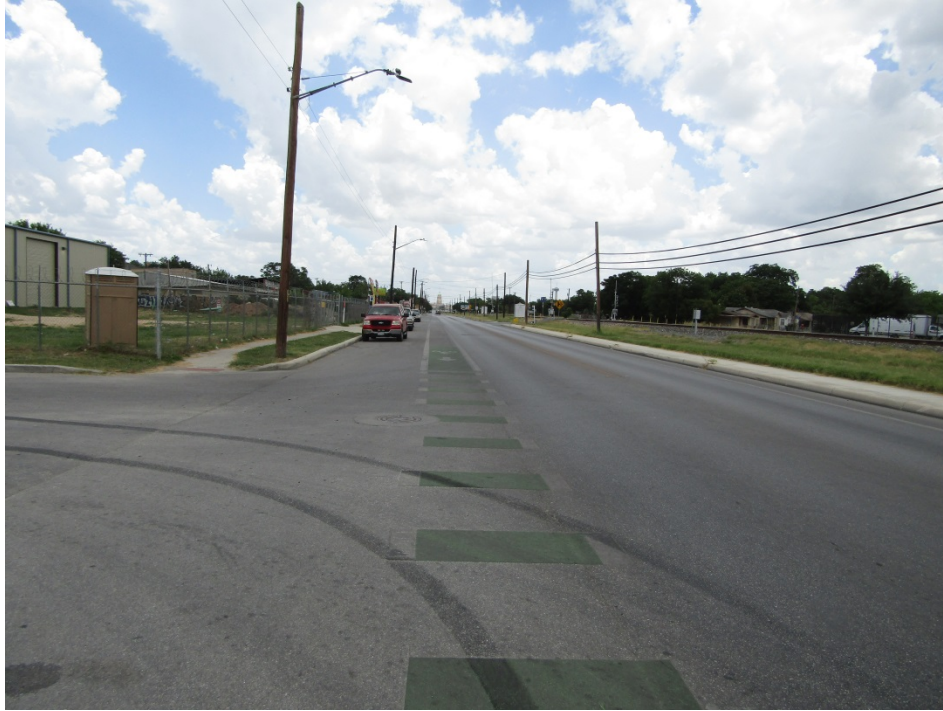
Streetscape Frio City Road (northeast)
