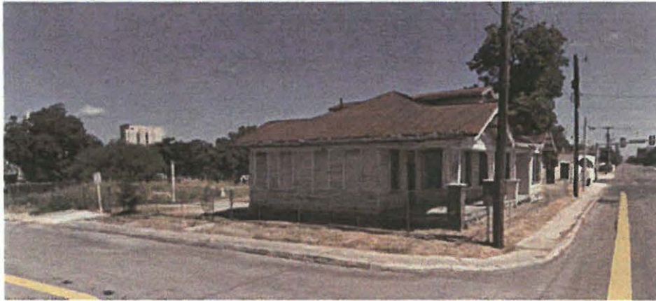
Residential structure located in the rear of 1434 E. Commerce parcel on the corner of Hackberry and Idaho.
