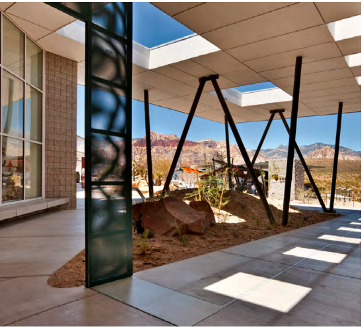
RED ROCK CANYON VISITOR CENTER: LAS VEGAS, NV
