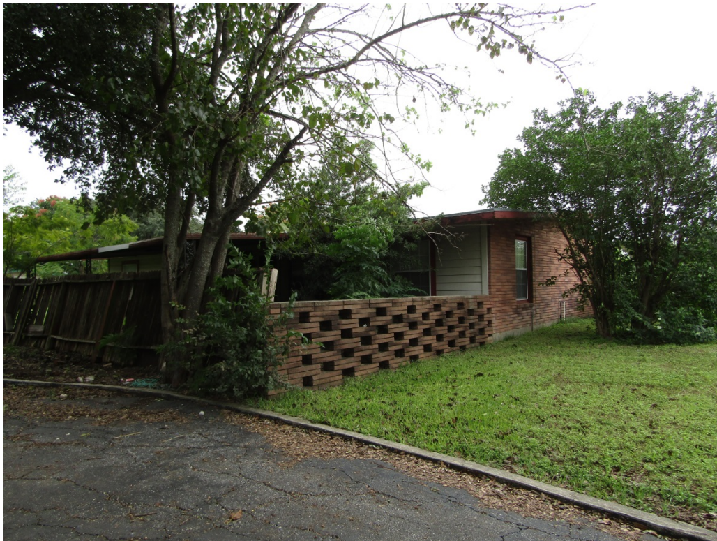
Neighboring Property (west)
