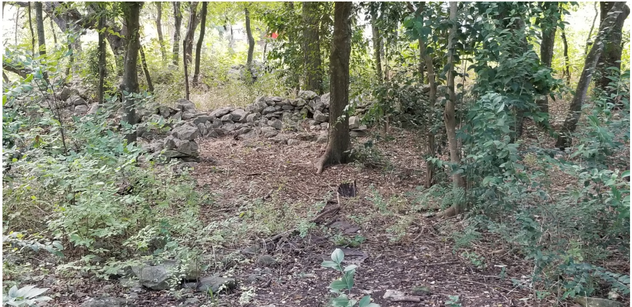
Low stacked stone walls found along the southern section of the property.
