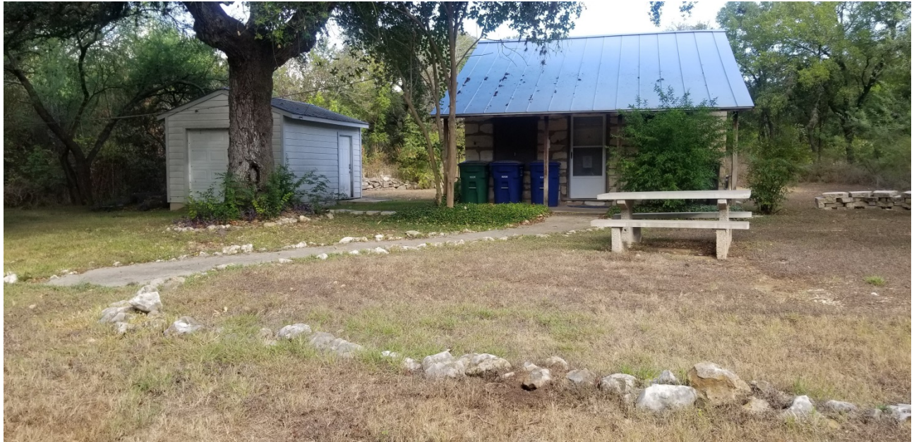
Primary façade and adjacent noncontributing modern garage.
