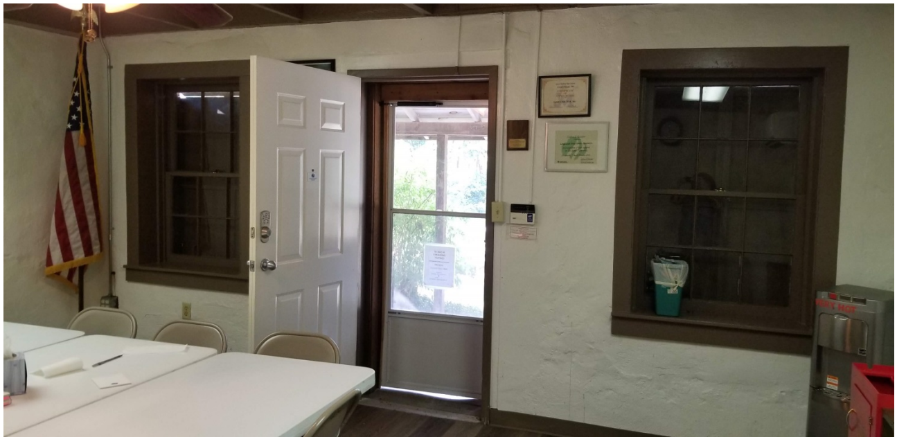
Interior view showing south-facing windows on primary façade, otherwise hidden by steel window gates.
