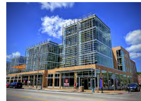
Developed by Washington University in St. Louis, Missouri, the Lofts of Washington University is a student housing and retail mixed-use project along a vibrant commercial corridor a 1/2-mile from the main university campus.
