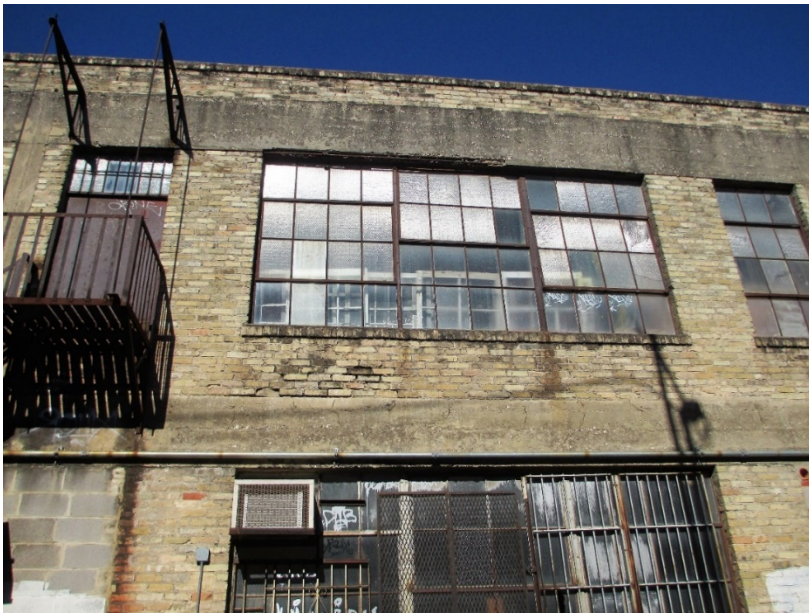
EAST - 2 ND FLOOR AT FIRE ESCAPE
