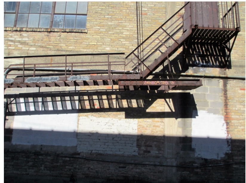
EAST - AT FIRE ESCAPE
