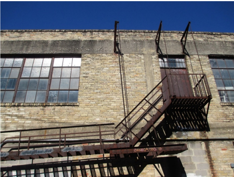
EAST - 2 ND FLOOR AT FIRE ESCAPE
