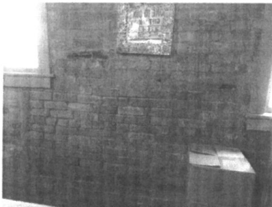
Building 21A—Brick wall
