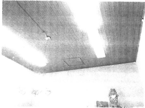
Building 3-Wood ceiling
