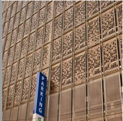
* Typical Architectural Installation of Perforated metal with varying hole sizes
