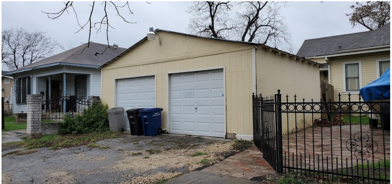
Garage, south and east elevations
