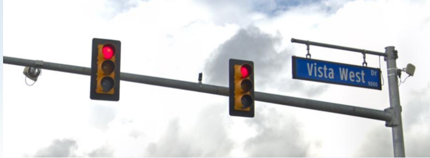
Steel Mast Arms, Vehicle Detection & ILSN
