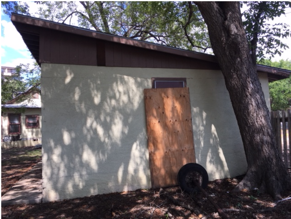
410 Barrera – Rear of Garage
