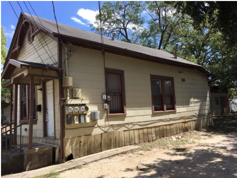
414 Barrera – West Side of House
