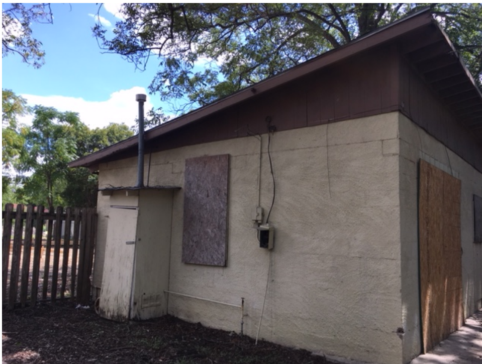
410 Barrera – Front of Garage (North)
