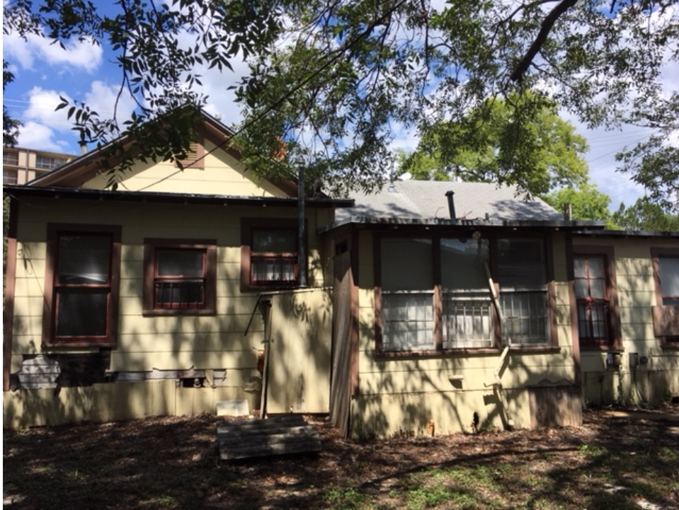
414 Barrera – Rear of House
