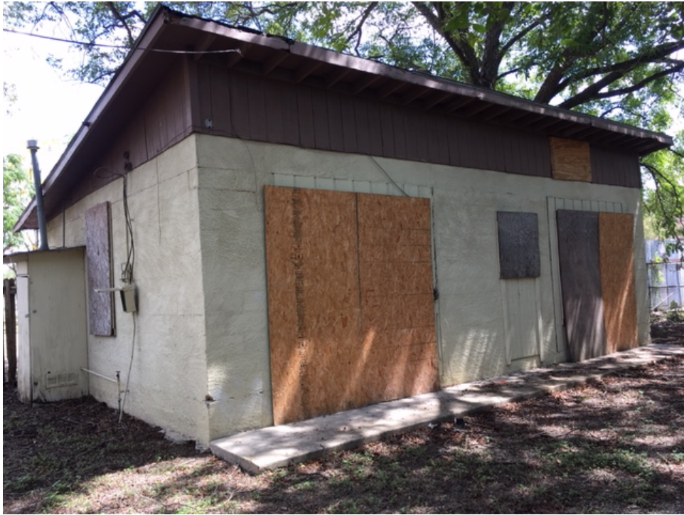
410 Barrera – West Side of Garage
