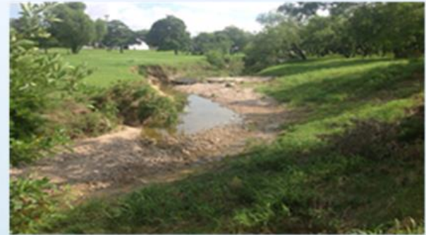
Bank Failure/Channel Widening
