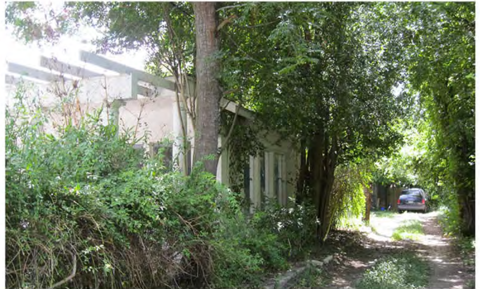
112 LINDELL PL. - EXISTING BUILDING / SIDE ALLEY OFF OF LINDELL PL.
