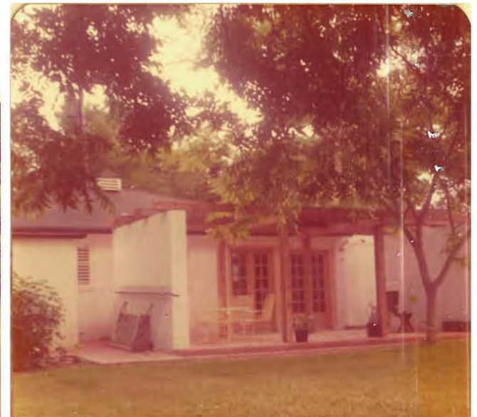
112 LINDELL PL. - BACKYARD PATIO ADDITION
