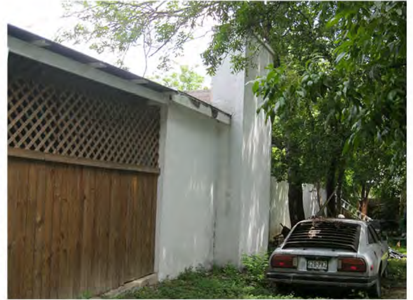
112 LINDELL PL. - EXISTING BUILDING VIEW FROM NEIGHBOR SIDE
