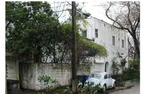
⑥ NE CORNER OF ARMOUR PLACE
