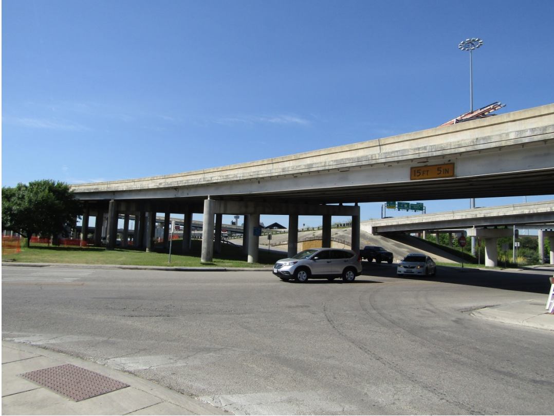
View across subject property
