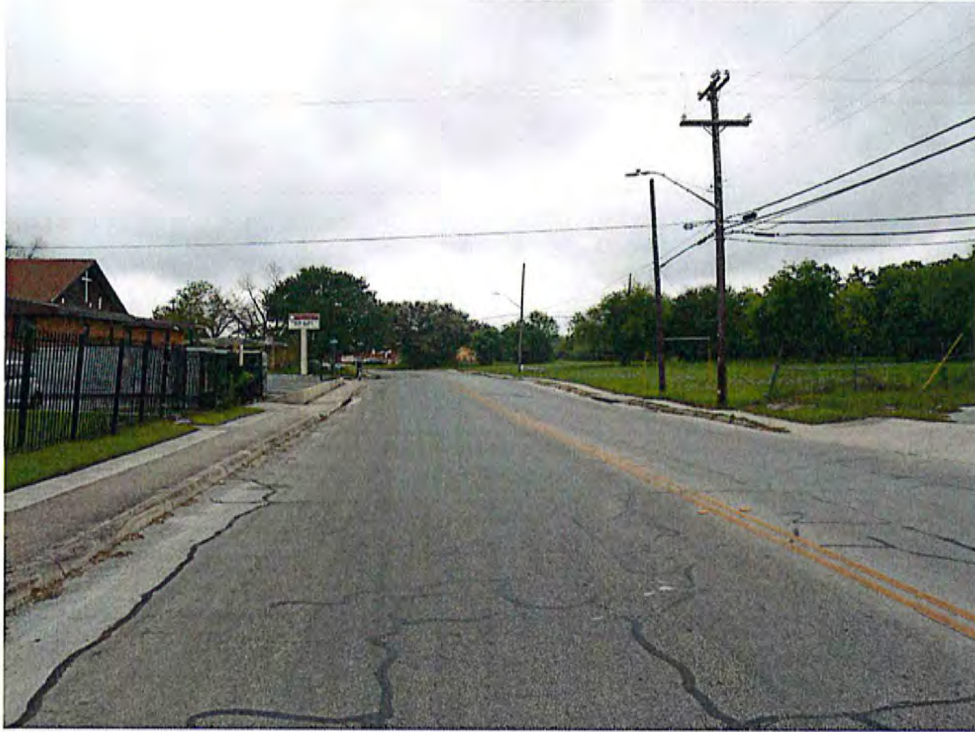
LOOKING SOUTHEAST ON SPRIGGSDALE AVENUE – SUBJECT AT RIGHT
