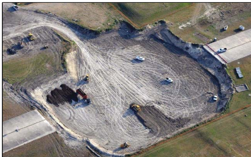
Airfield Projects at San Antonio International Airport
