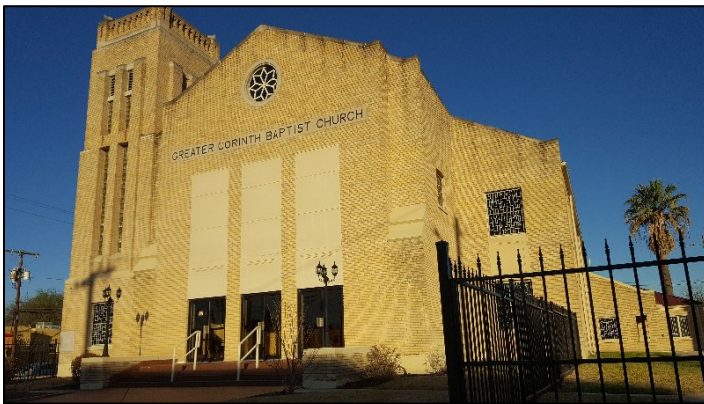
508.518 S New Braunfels Ave – Greater Corinth Baptist Church
