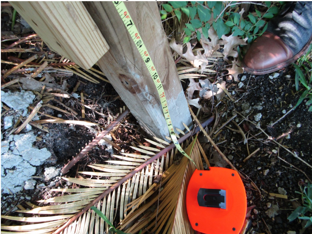
Height of replaced fence
