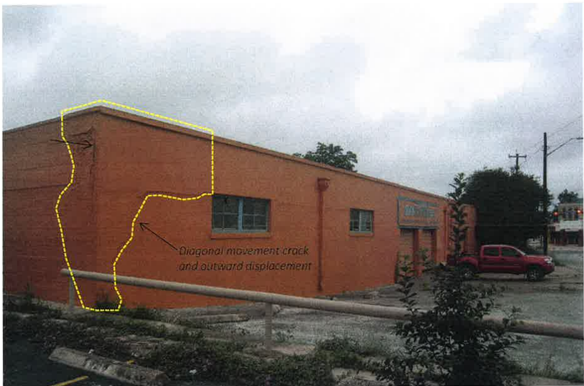
Figure 4: Cracking at the southeast corner along horizontal datum of the lintels and concrete frame.
