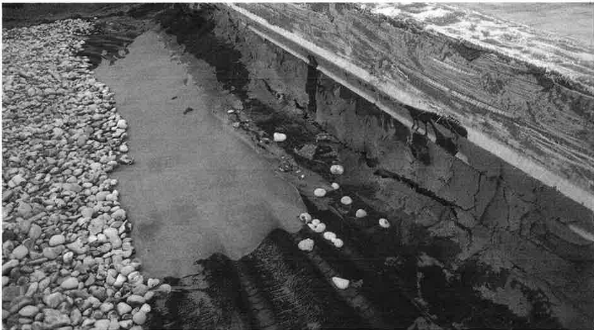
Figure 6: Drainage inadequacy is causing water to pond on the roof.
