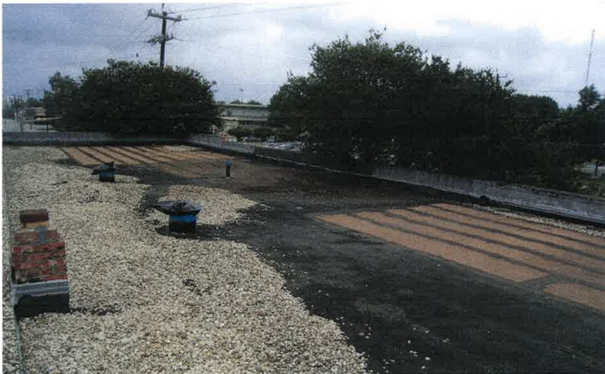
Figure 2: Drainage inadequacy from tree foliage above roof.
