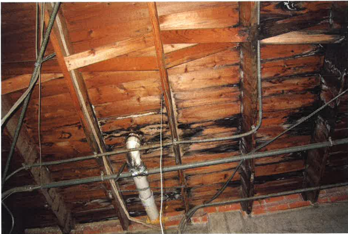
Figure 3: Deterioration of the roof deck and framing below poor roof drainage.
