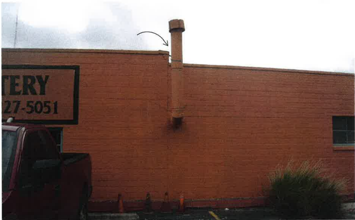
Figure 5: Loose parapet masonry at the vent roof tie-back.
