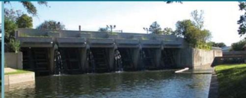
SAN ANTONIO RIVER TUNNEL INLET
