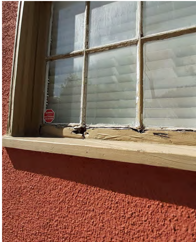
Images of the windows starting at the corner of Beauregard St and Madison. As can be seen, many of the windows have not been maintained properly over the years. - co in many areas. The Residence renovation is in Unit 2; 2nd Floor Apartment (directly above thee 222 plaque. Window 2, with missing Rail overlooks this sidewalk.
