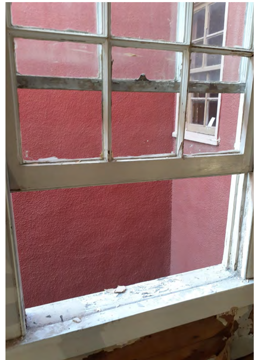
Window does not stay open for long, it slowly lowers on its own.
