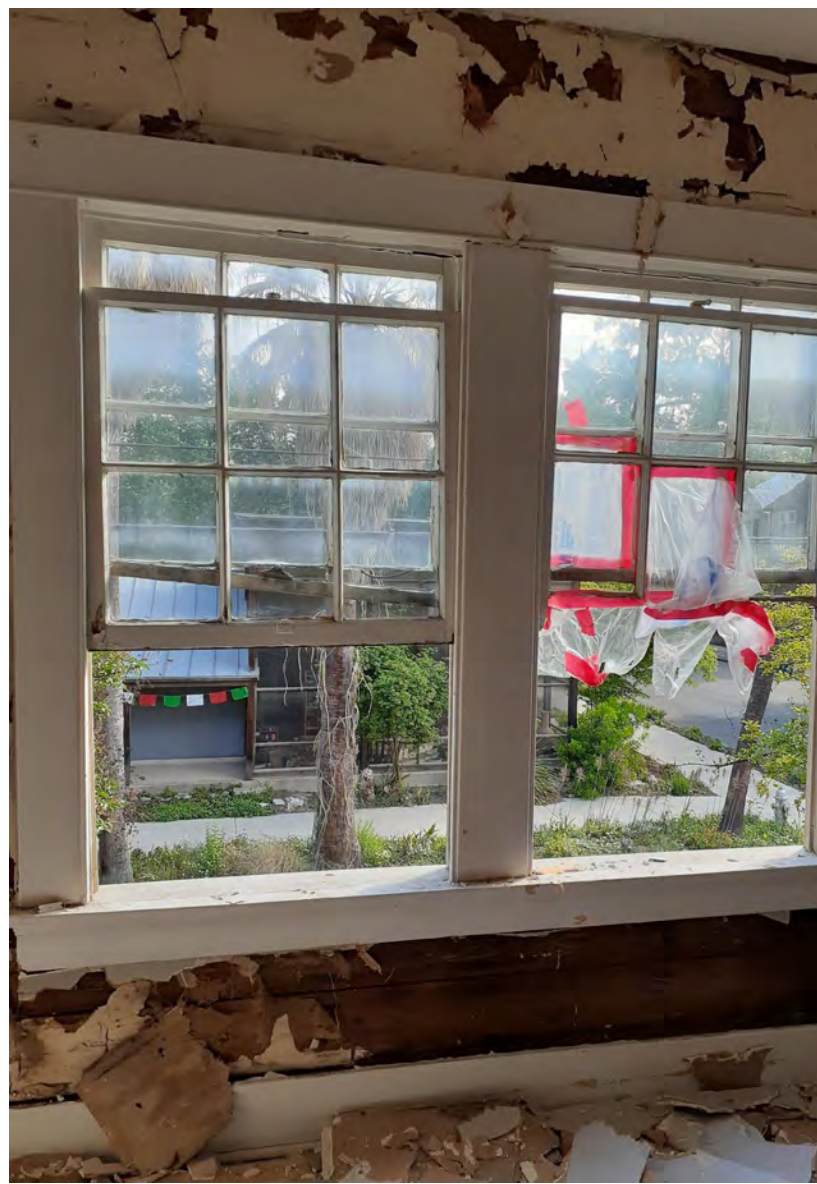
Overall Window 2: Multiple layers of paint and caulk over water damaged wood, typical.
