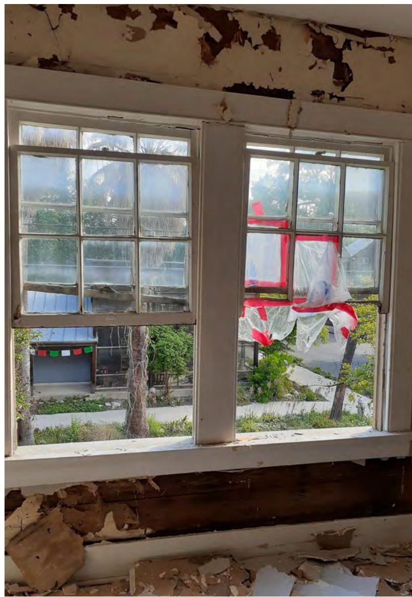
Overall Window 3: Multiple layers of paint and caulk over water damaged wood, typical.
