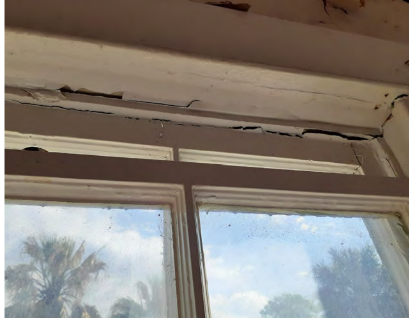
Overall Window 3: Multiple layers of paint and caulk over water damaged wood, typical.
