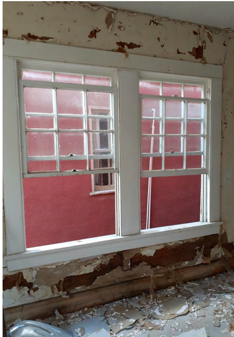
over water damaged wood, typical.
