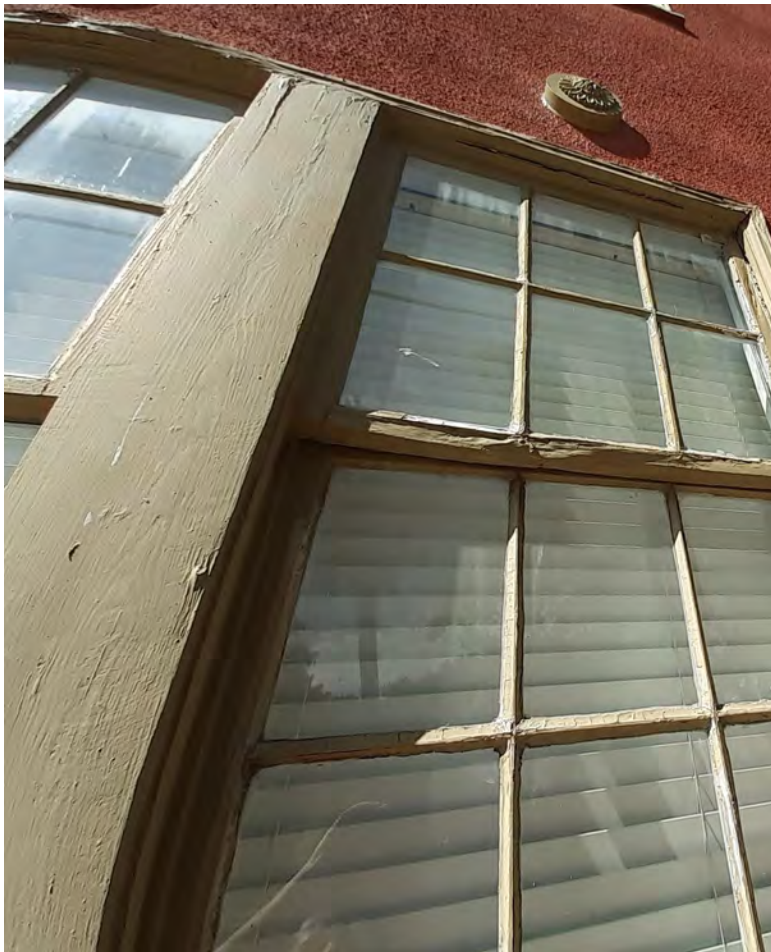
Images of the windows starting at the corner of Beauregard St and Madison. As can be seen, many of the windows have not been maintained properly over the years. - co in many areas. The Residence renovation is in Unit 2; 2nd Floor Apartment (directly above thee 222 plaque. Window 2, with missing Rail overlooks this sidewalk.
