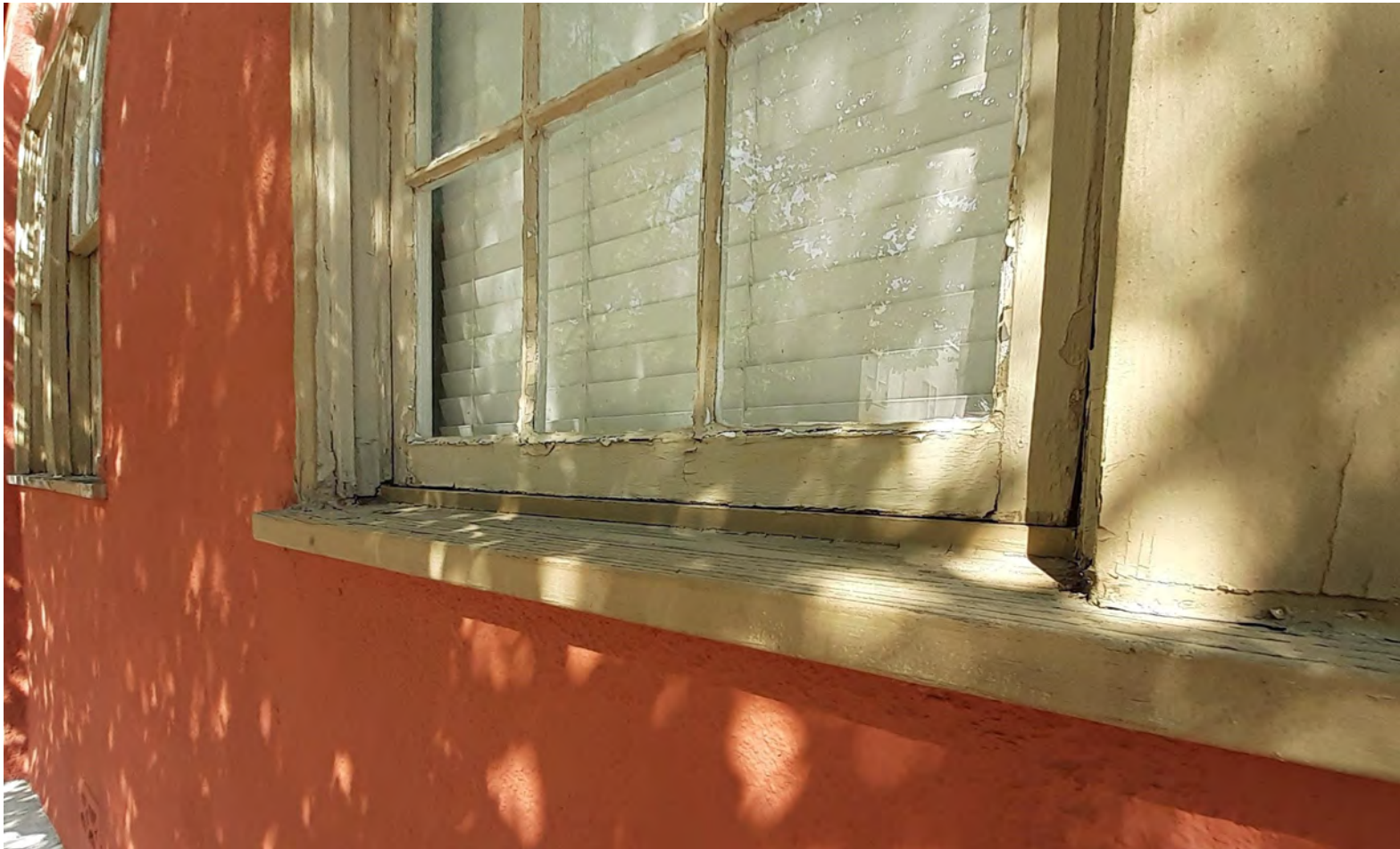
Typical Window condition, extensive water damage and aging has occurred.
