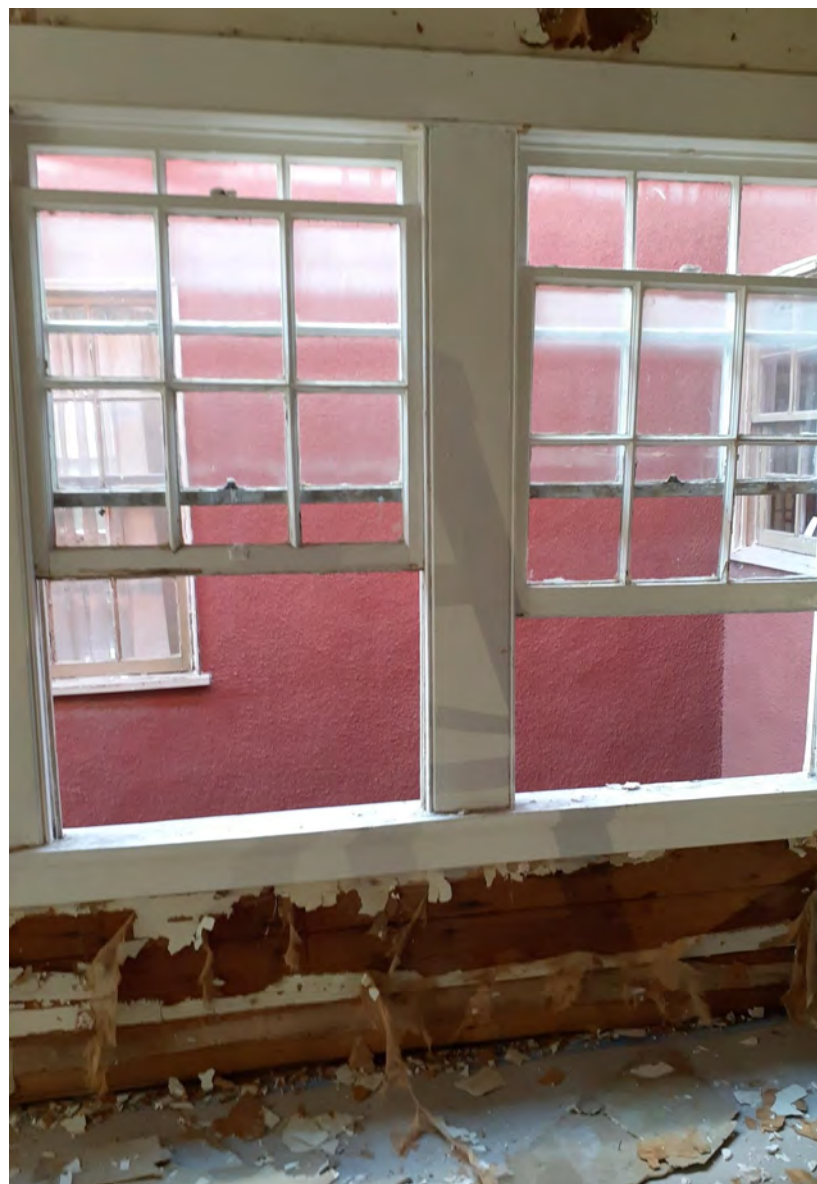
over water damaged wood, typical.
