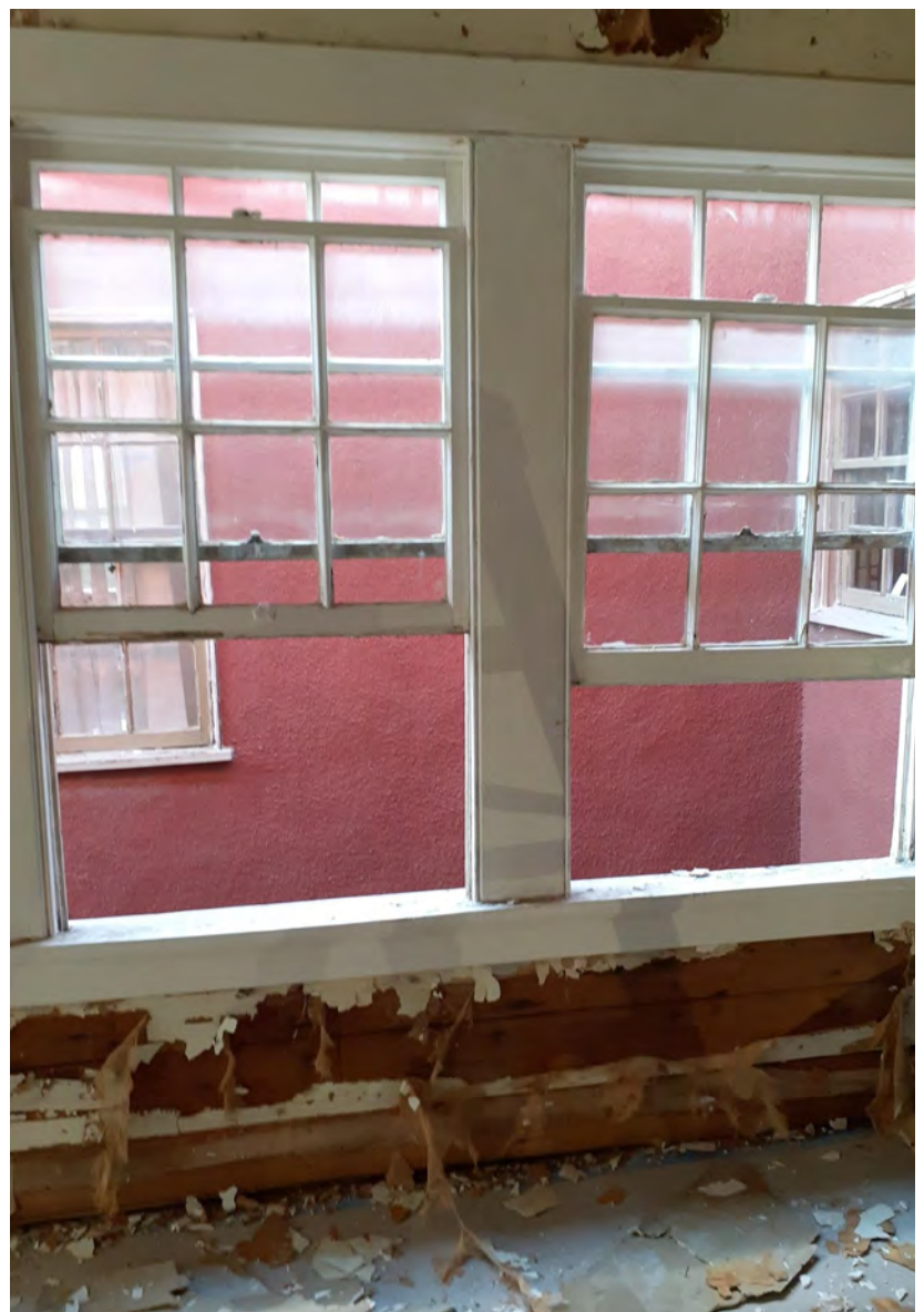
Overall Window 7: Multiple layers of paint and caulk over water damaged wood, typical.
