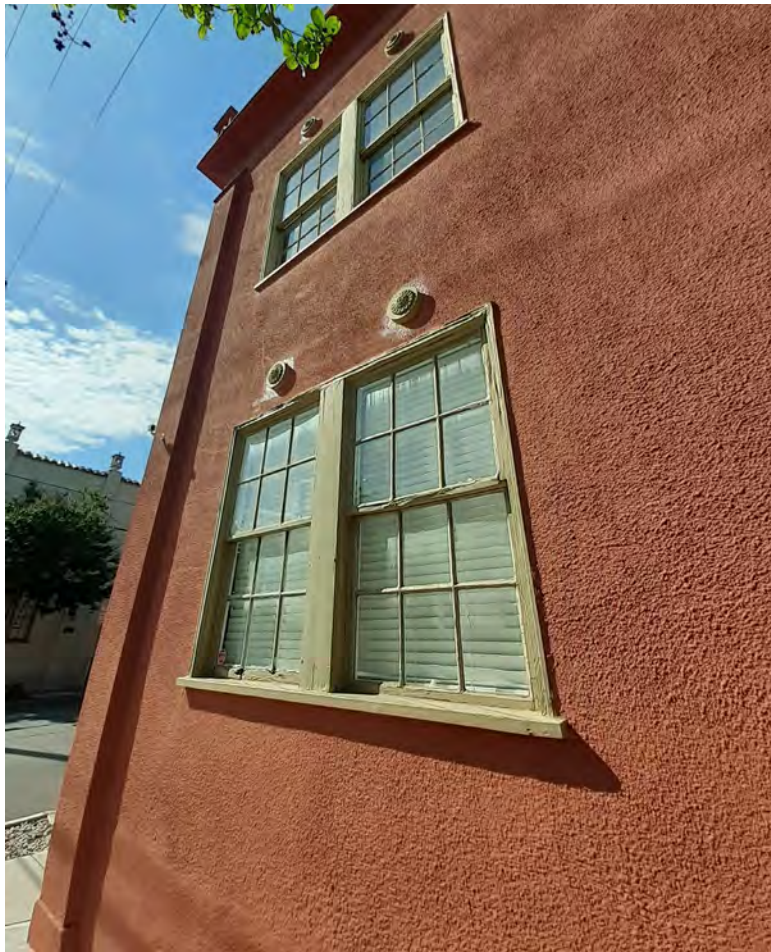
Images of the windows starting at the corner of Beauregard St and Madison. As can be seen, many of the windows have not been maintained properly over the years. - co in many areas. The Residence renovation is in Unit 2; 2nd Floor Apartment (directly above thee 222 plaque. Window 2, with missing Rail overlooks this sidewalk.
