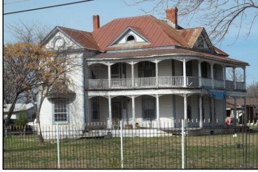
Two Story House 4527 W. Martin
