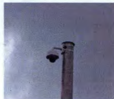
Traffic Monitoring Cameras
