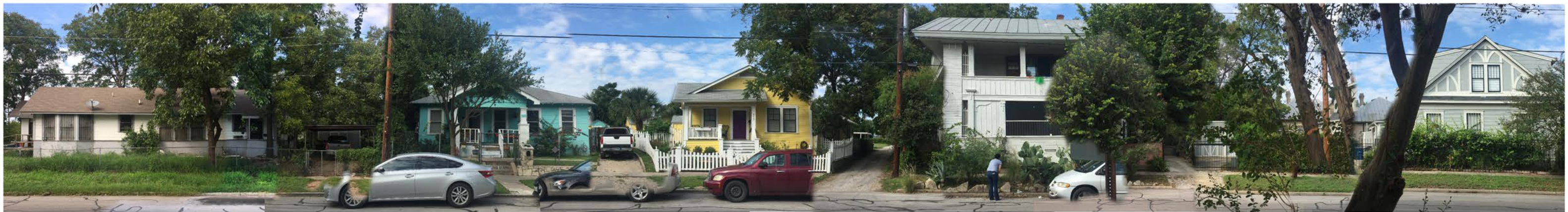
Burnet Street elevation - north side
