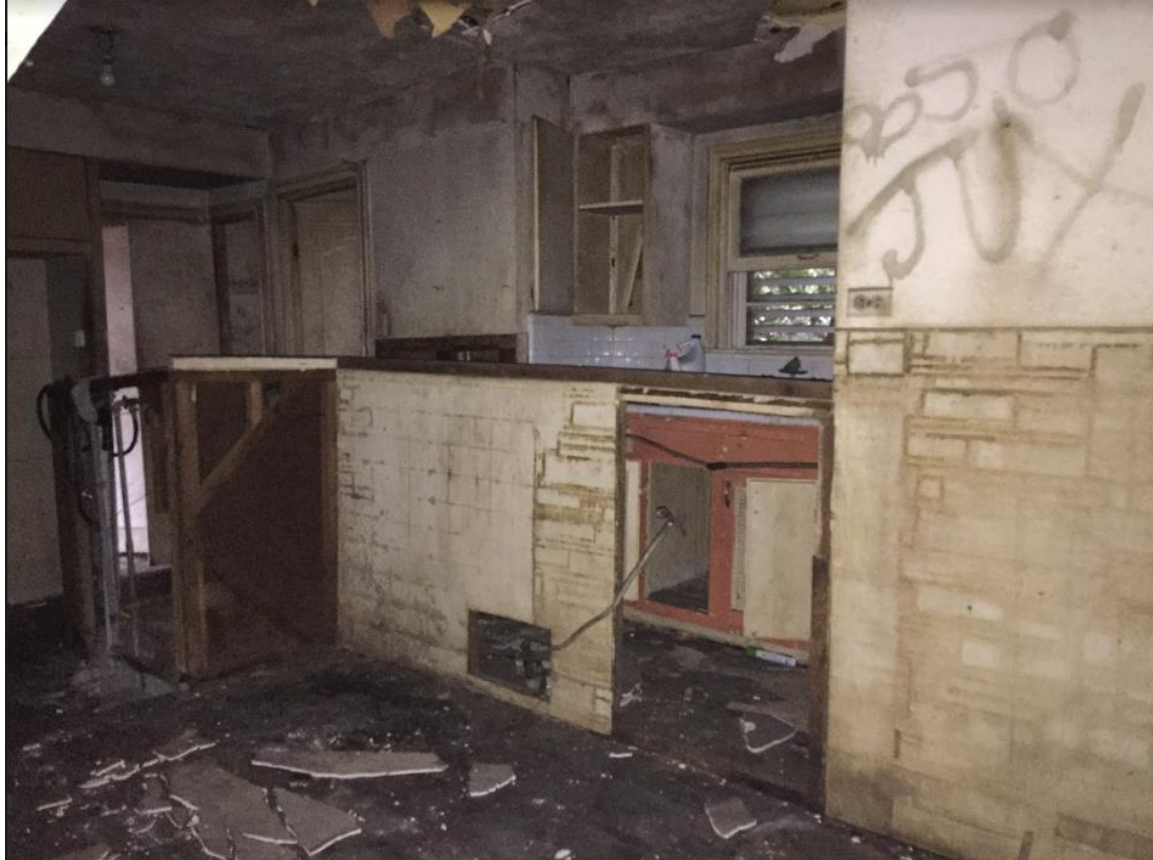
205 Ostrom Drive Interior Photo's 23 Years Abandoned
