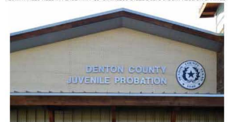
6" ALUMINUM SEAL WITH 3" RETURN AND PRECISION CUT ALUMINUM LETTERS
