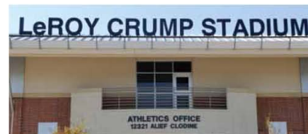
30" LETTERS, FABRICATED ALUMINUM, 3" THICK
