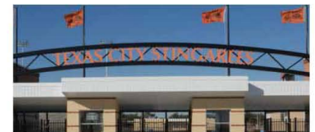
24" PAINTED PRECISION CUT ALUMINUM LETTERS, 1/4" THICK
