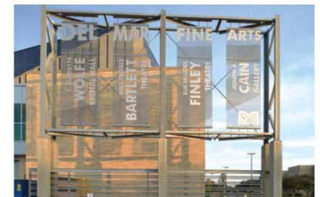
1/8" THICK PRECISION CUT ALUM. MECHANICALLY MOUNTED TO TWO 15' X 5' PERFORATED ALUM. PANELS HELD IN PLACE WITH 1/2" STAINLESS STEEL BOLTS & COMPRESSION SPRINGS
