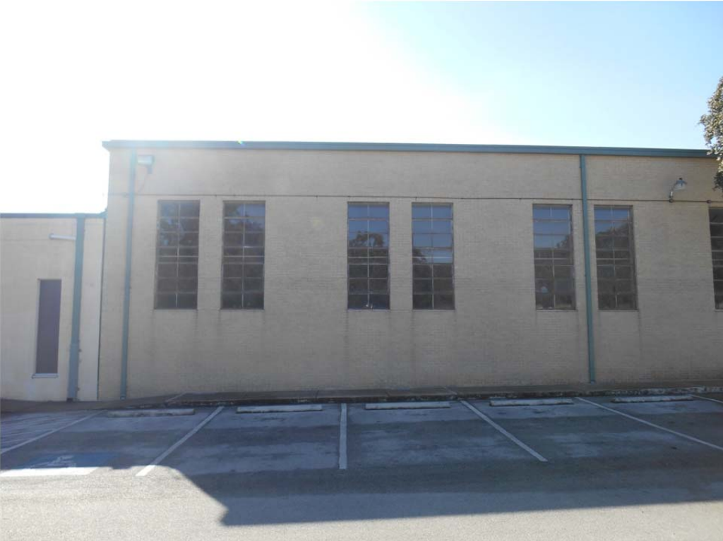
Figure 6 - Exterior of Gymnasium Windows
