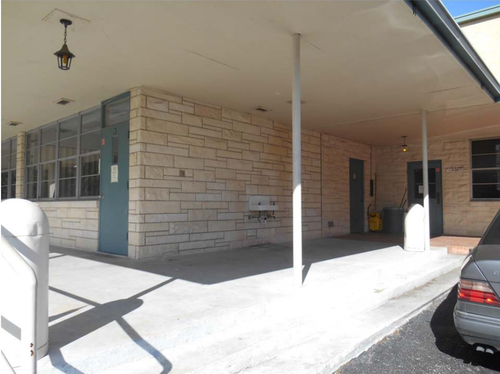
Figure 3 - Existing Covered Walkway
