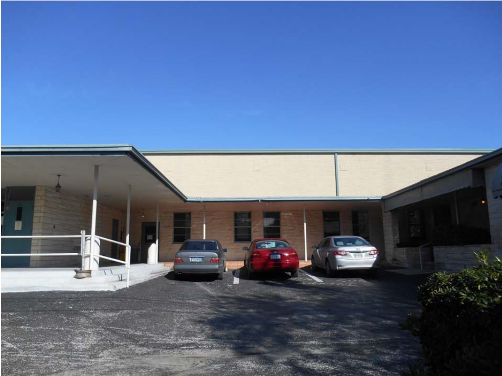
Figure 2- Existing Parking outside of Madonna Room
