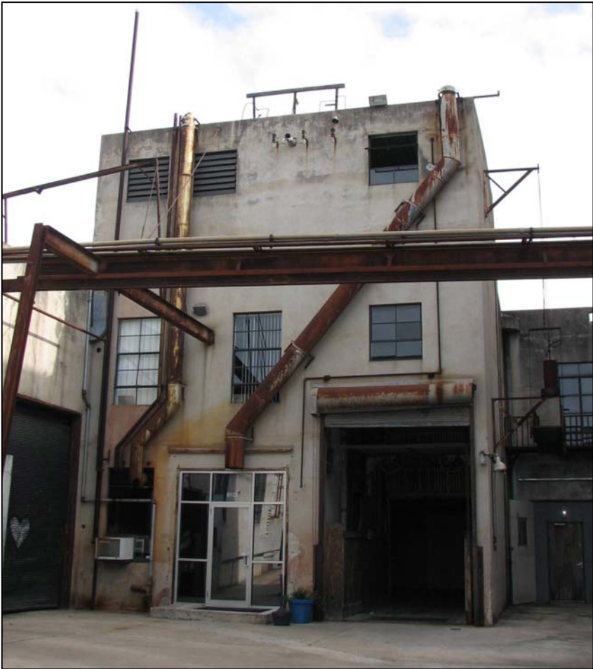
Infill Construction (1948) – between buildings 7, 10, and 11 – CONTRIBUTING
