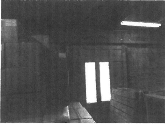
Building 21A—Storage and loading
