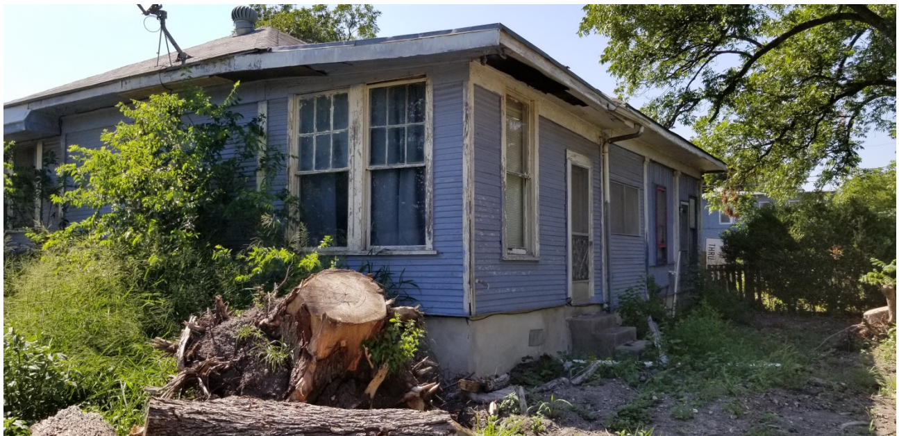
Rear (south) and east elevations
