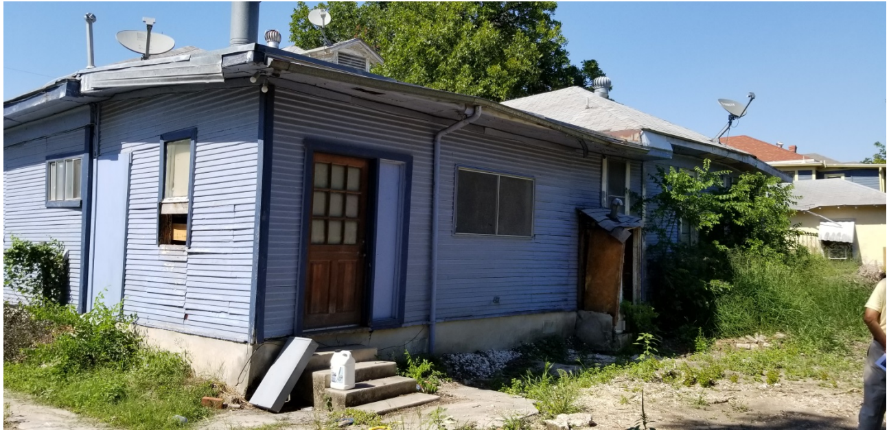
Rear (south) and west elevations
