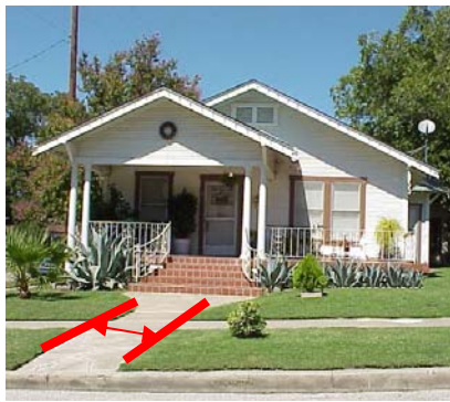
Typical example of front walkway on a residential property; Single-family structures require a 3 foot walkway
