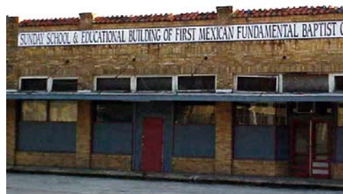
Non-conforming example of a commercial building that has window and door openings that have been partially covered with non-transparent materials
