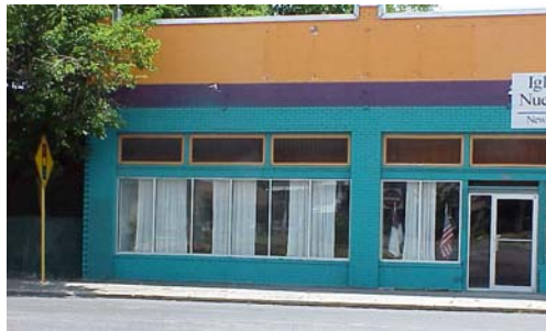
Example of conforming window and door openings on a commercial structure
