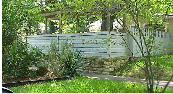
Examples of non-conforming fences in front yard
