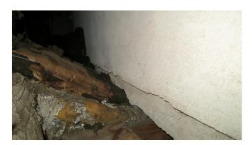
Figures 22 and 23: Traces of plaster indicate the middle area of the house was lowered by the Swans in the 1960s.
