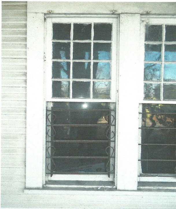
(WINDOWS DESIGNATED TO REMAIN) EXISTING WOOD WINDOWS ON THE HOUSE
