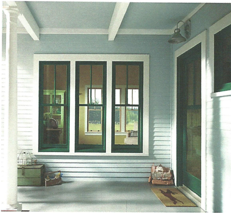
EXTERIOR PHOTO/EXAMPLE OF ANDERSON COMPOSITE (WOOD & VINYLE) "FIBREX" SINGLE HUNG WINDOW FRAME WITH WOOD TRIM ON WOOD SIDING
