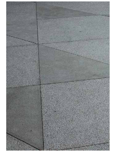
Upgraded vehicular concrete
