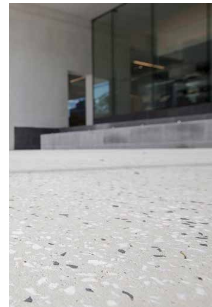
Upgraded pedestrian concrete
