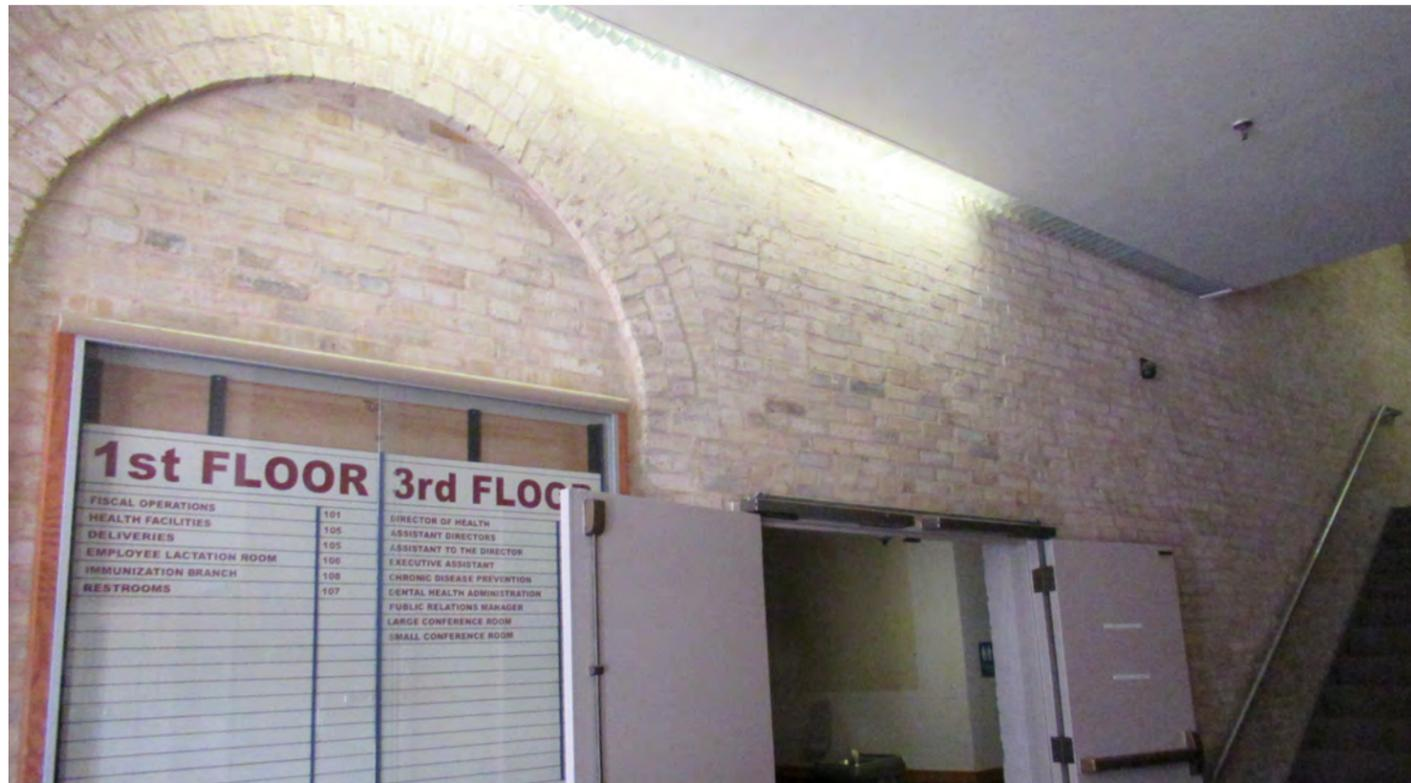
First floor interior showing original masonry bearing wall & non-historic stair
