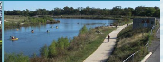
SAN ANTONIO RIVER – ESPADA PARK
