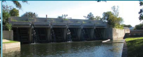
SAN ANTONIO RIVER TUNNEL INLET
