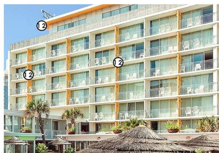
CURRENT CONDITION OF YELLOW PAINT
