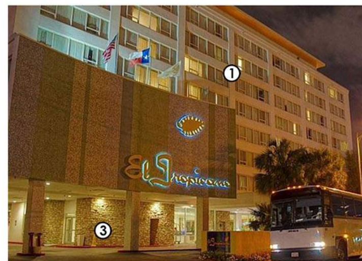
CURRENT CONDITION WITH STUCCO AND STONE
