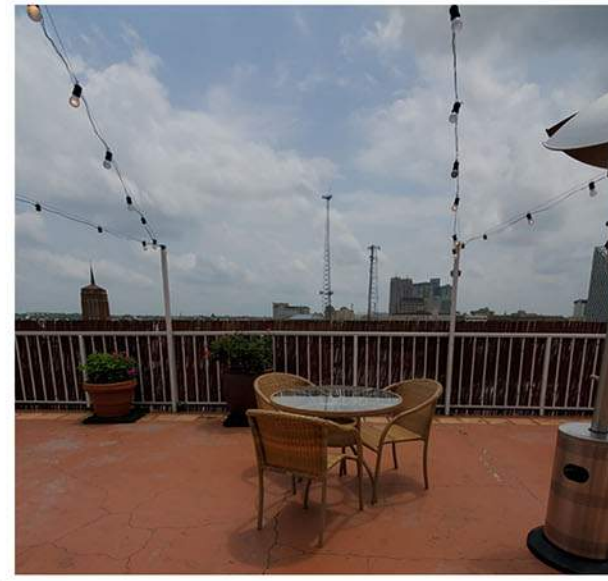
EXISTING BAMBOO RAILING
