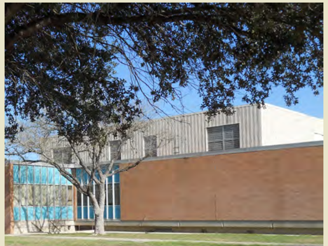
Mechanical equipment located on the roof of a building to hide it from direct view.
