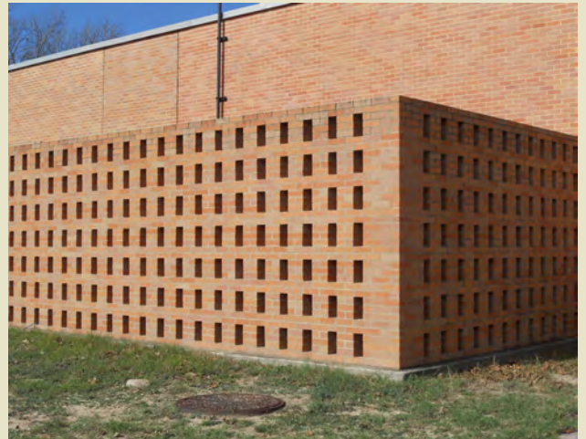
Mechanical equipment screened behind a patterned brick wall.
