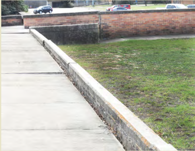
Retaining walls used on the campus to deal with changes in topographic elevations.
