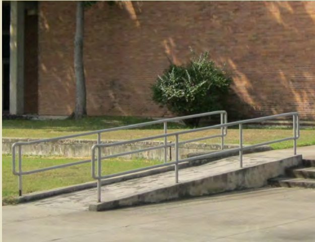
Accessible ramp leading to the library. Does not interfere with the historic facade or character because of placement.
