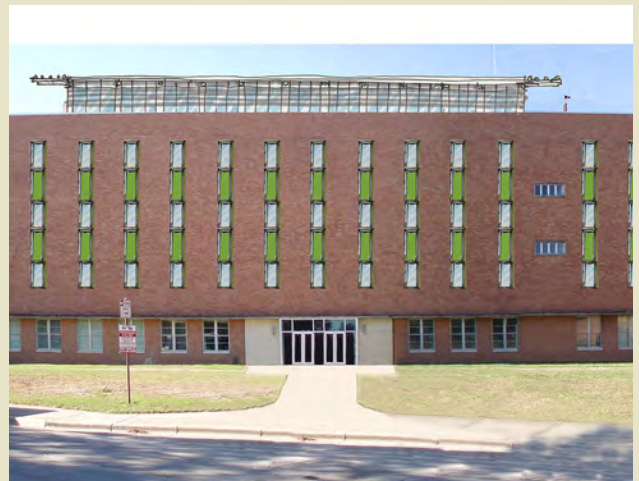
Roof additions can be modified as clerestories and light wells.
