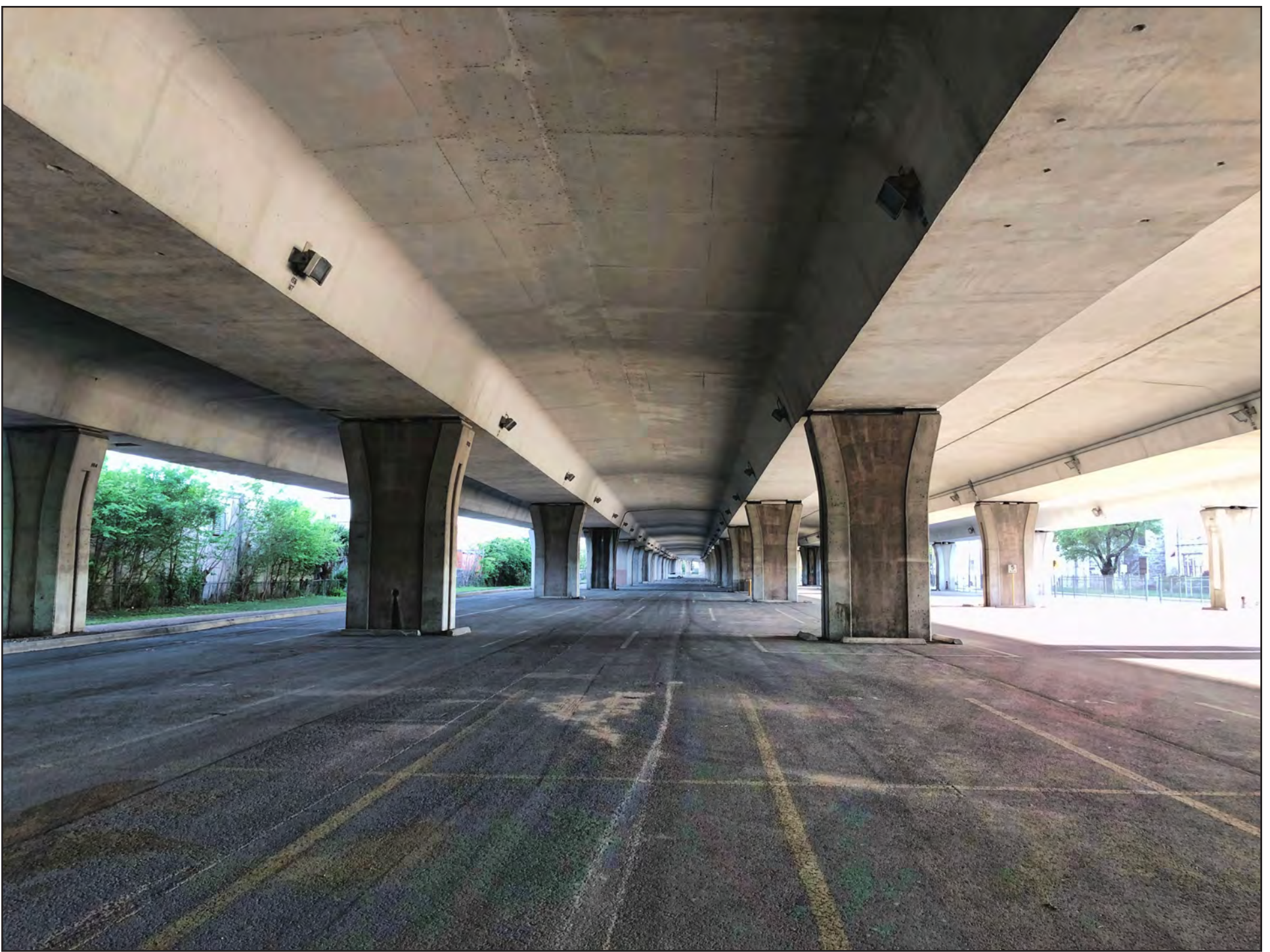
[Figure 22] - Underpass Lighting - Existing
